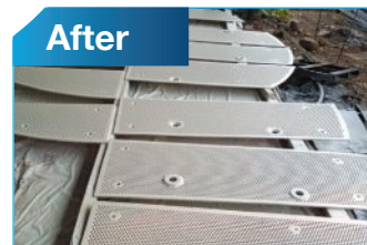
Filter bed bottom plates
