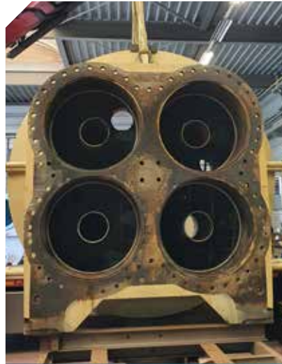
Cooling water area before protective coating
